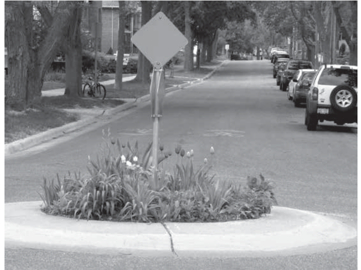
A traffic-calming island at Kendall and Grand Avenues
