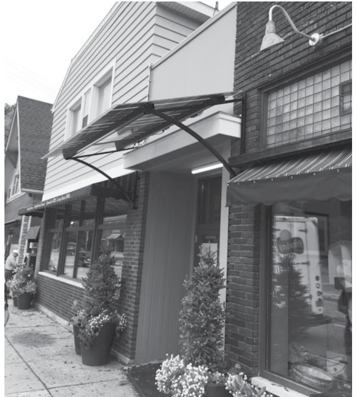
Regent Market Co-op's recently-installed solar awning
